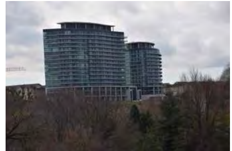
Scenic – Aspen Ridge Development located along the south side of Eglinton Avenue East at Brentcliffe Road
