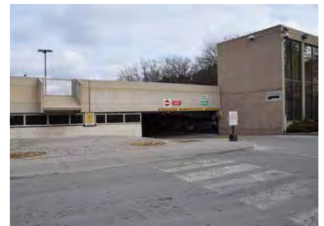
Parking garage used for the storage of vehicles located east of the Carrington Condominiums
