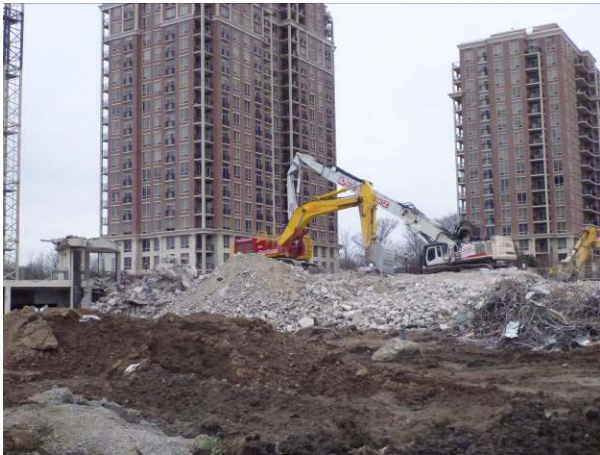
Plate 5: View of demolition area.
