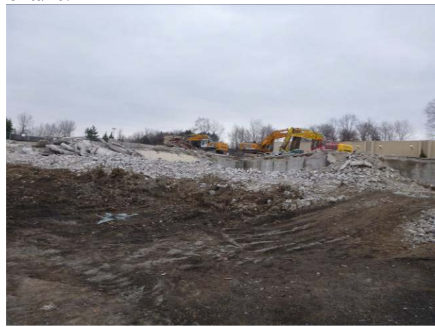
Plate 4: View of demolition area.
