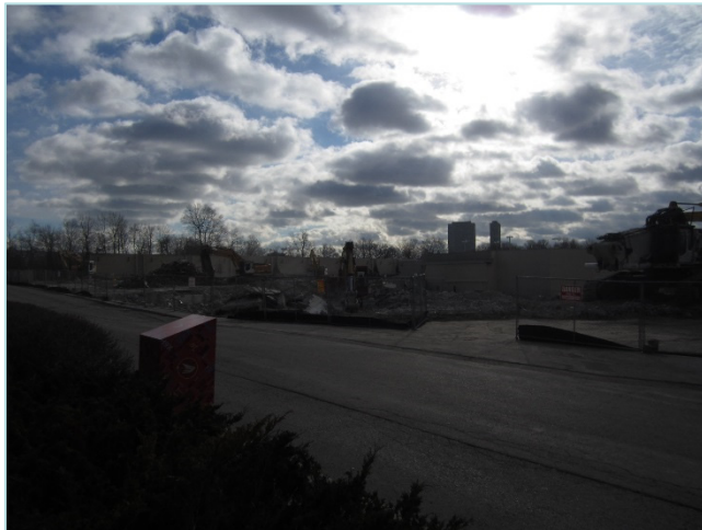
Figure 2a: Looking south at existing site
